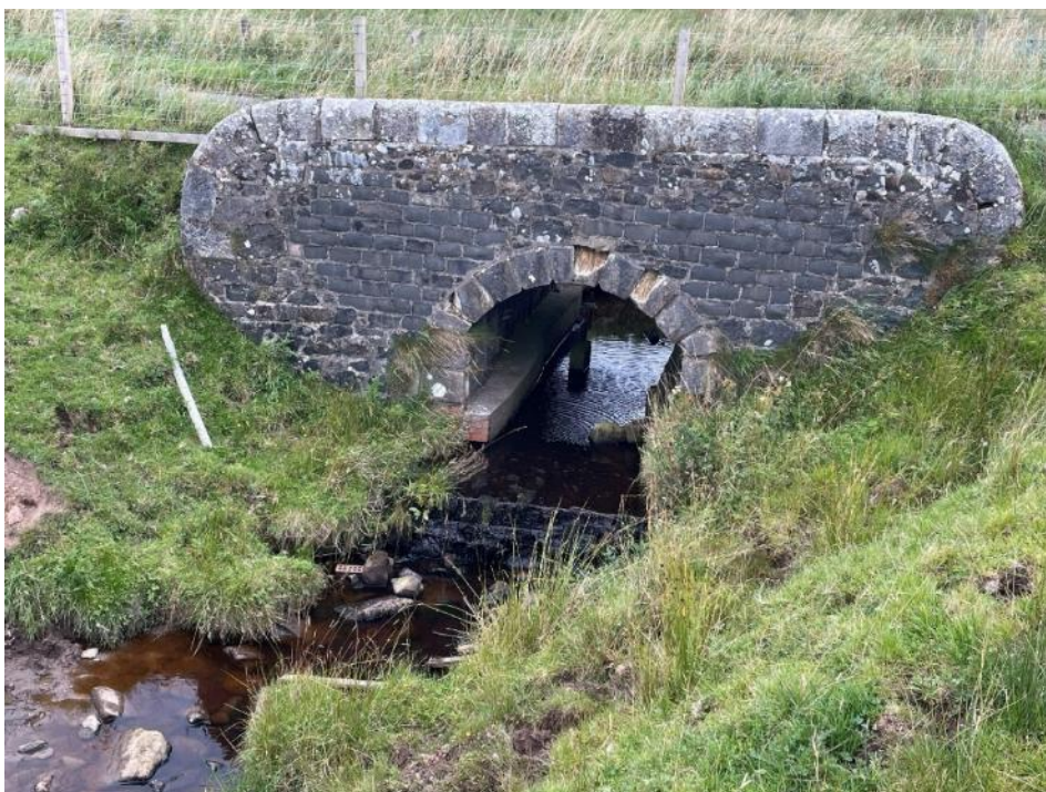
Photo 8: Small Burn - Road bridge apron preventing upstream migration
