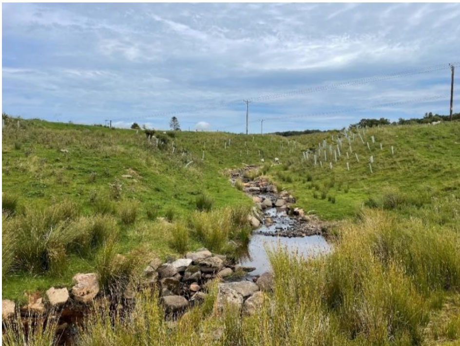
Photo 23: Boghead Burn - Looking upstream to the realigned river channel
