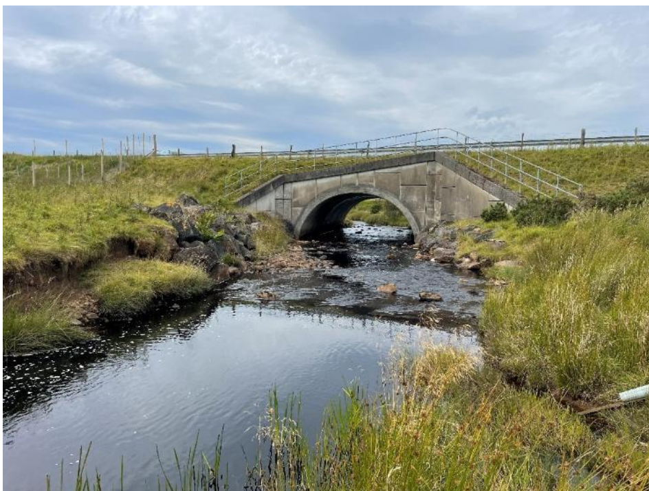
Photo 36: Gass Water - Lower limit of the habitat survey, confluence with the Boghead Burn and passable road culvert
