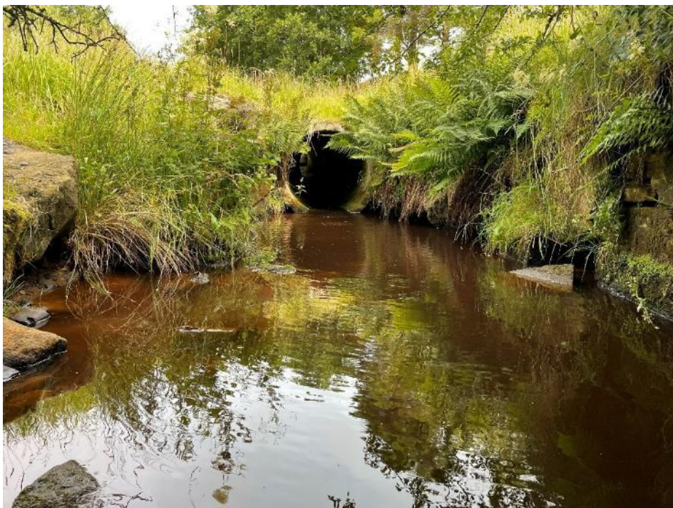
Photo 13: Glenmuir Burn - Large culvert
