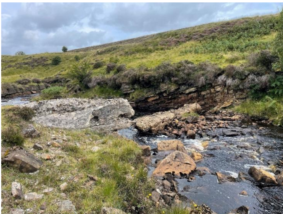
Photo 30: Gass Water - Remnants of the historic weir
