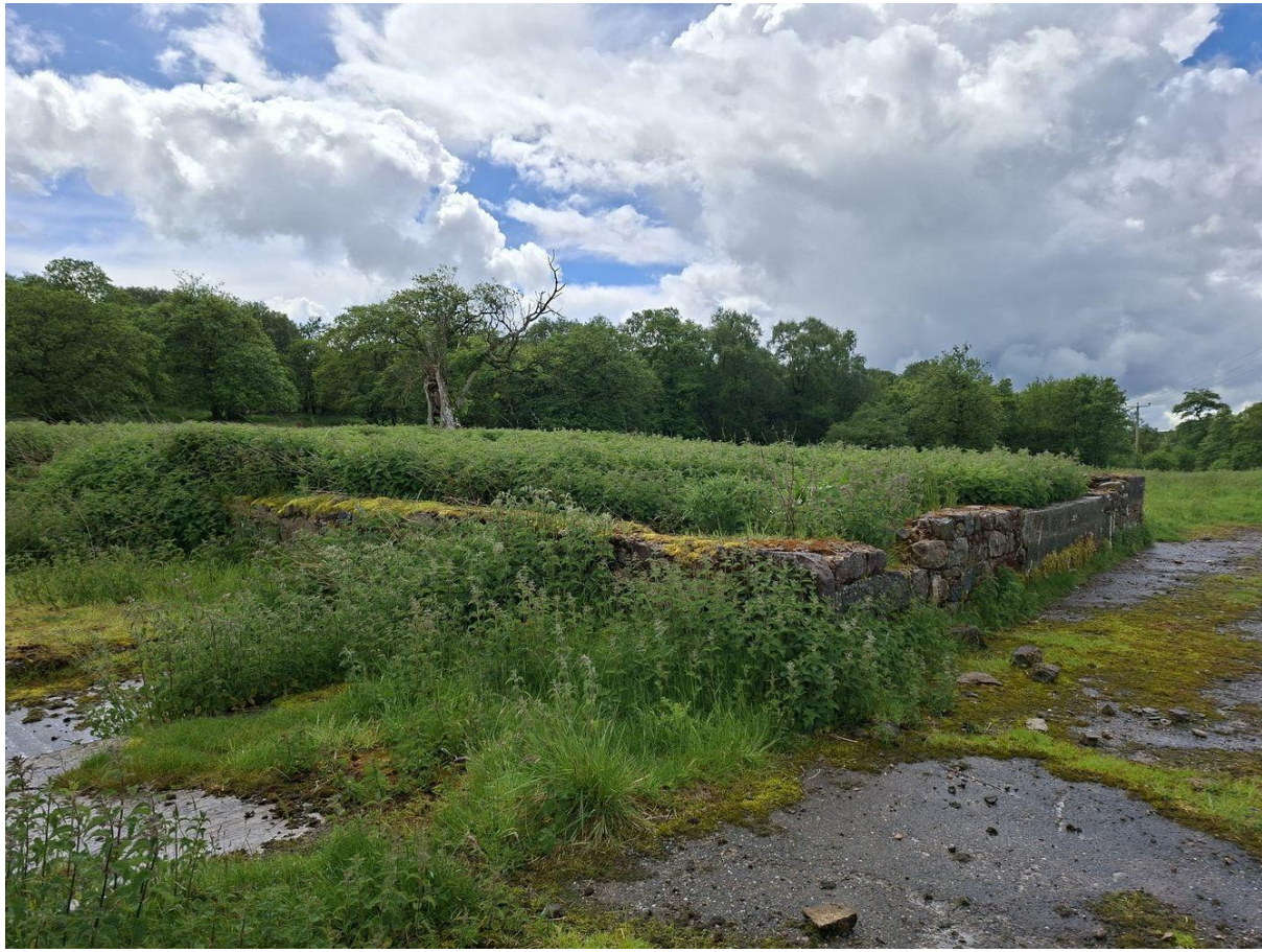
Photograph 1: Photograph of wall footings associated with SLR59.
