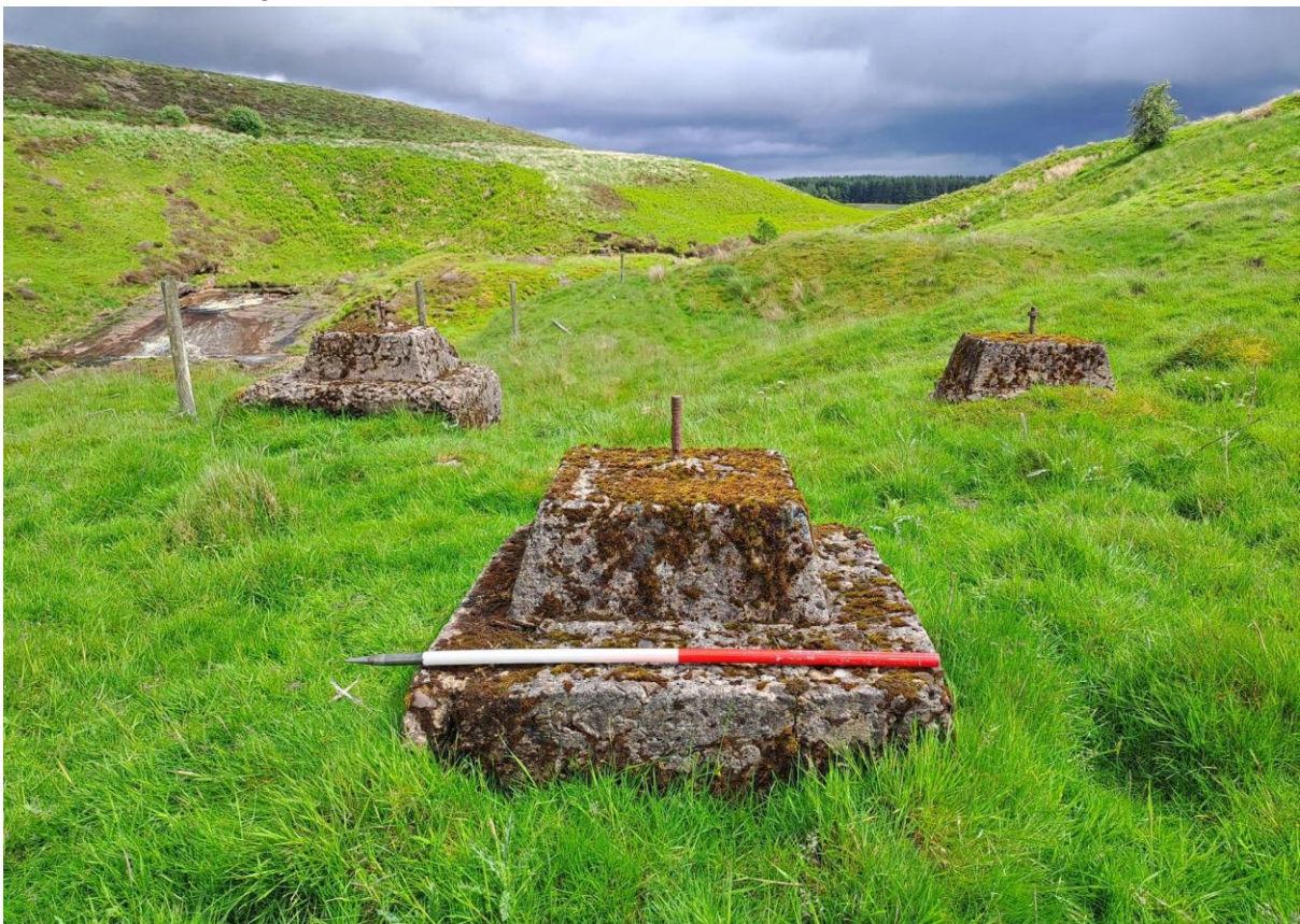
Photograph 2: Photograph of concrete footings associated with the aerial ropeway (SLR71)
