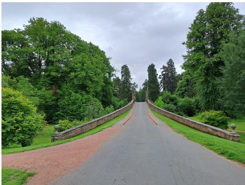
Photograph 11: View of LB14414 on approach from north
