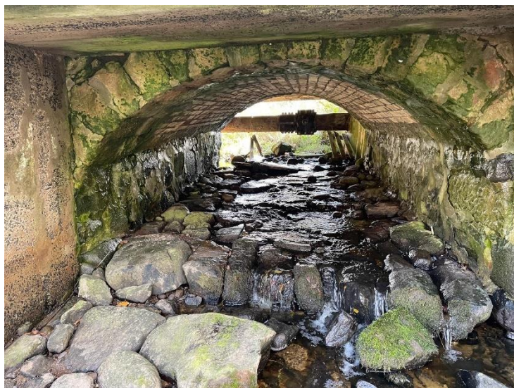
Figure 29: Site ABWUNB2 - Upstream limit of site - Bridge apron likely acts as a barrier under low and medium flow conditions
