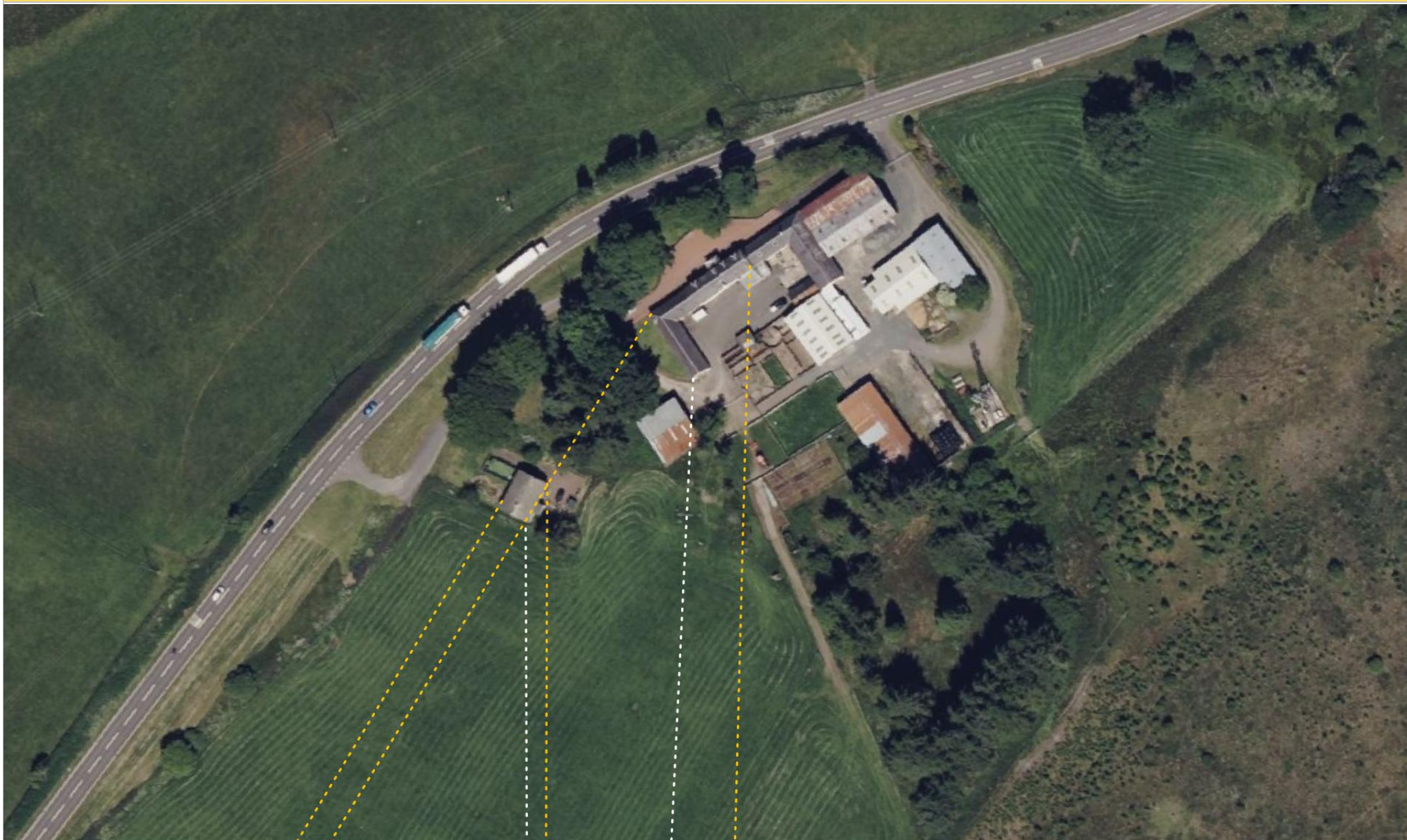
P1: Boghead Farm & P2: Dalvene Cottage – Aerial View
